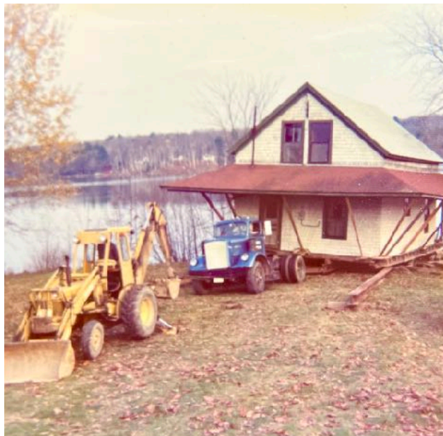
Heron House being moved off Pleasant Point to higher ground.
