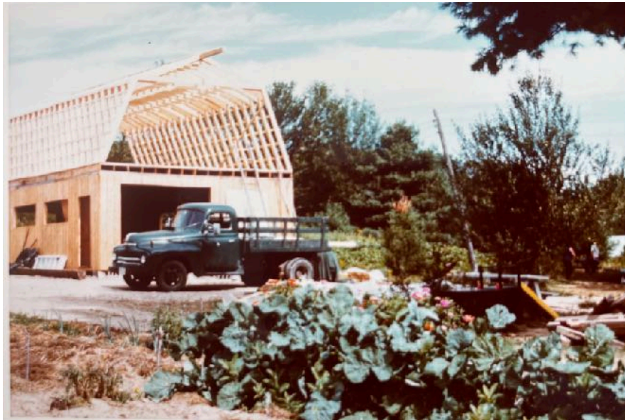
Sunshine Farm barn under construction in 1975.
